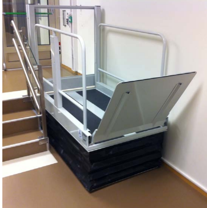
Public access lift with upper gate and control pillar
